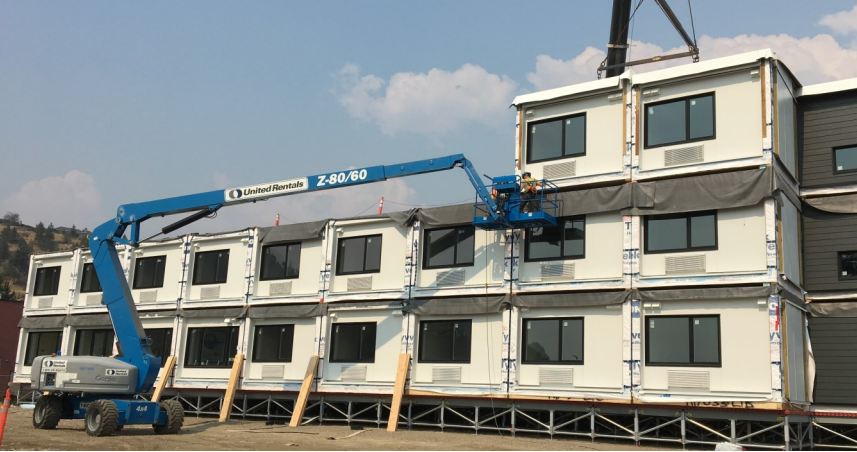
Kelowna, BC — 3 story housing project
